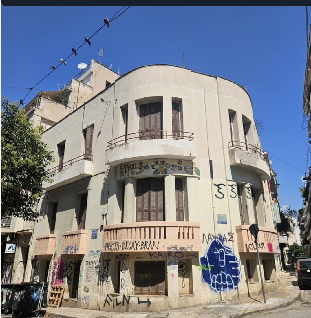
BEFORE - EXISTING CONDITION
