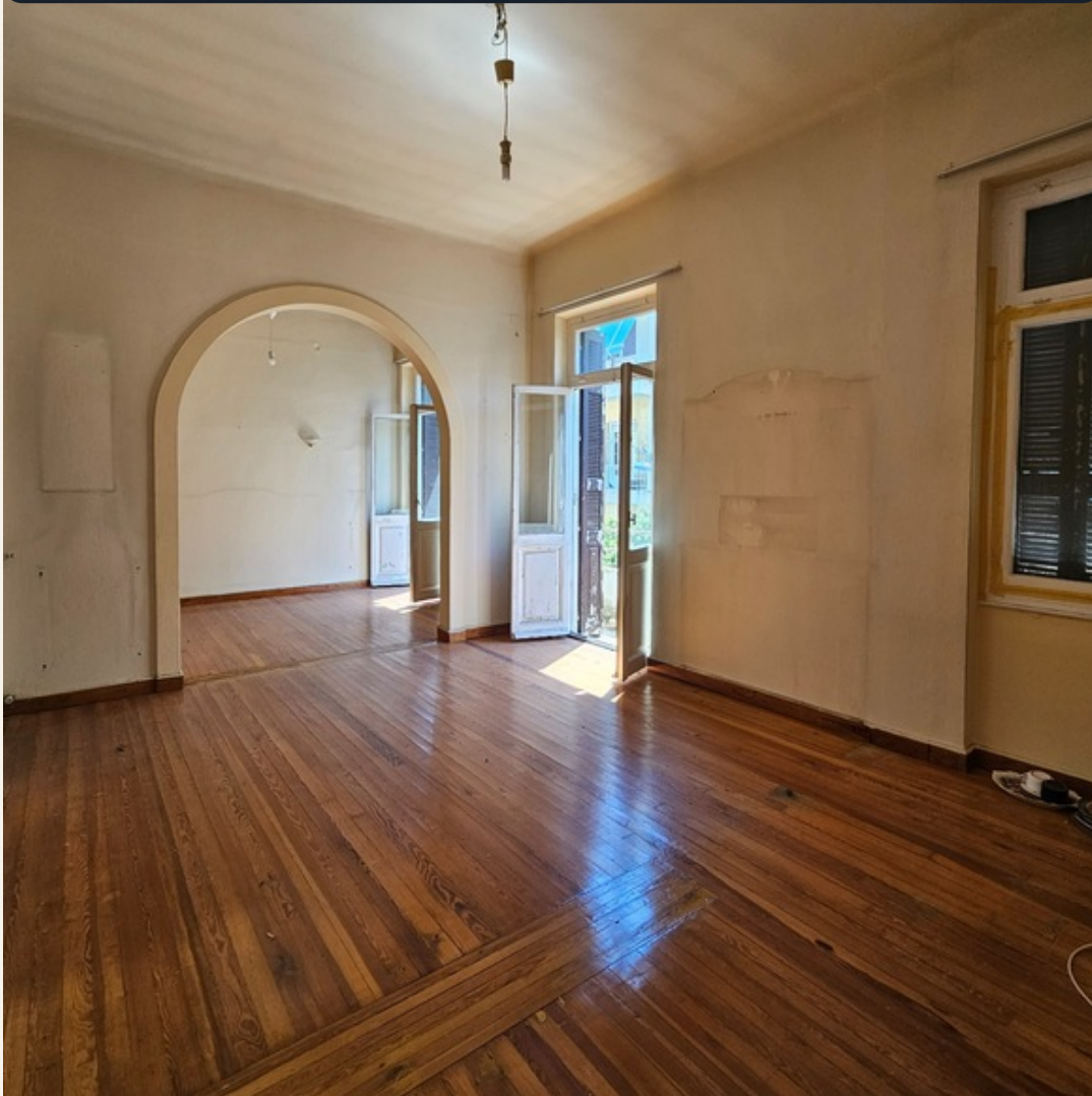
BEFORE - EXISTING INTERIOR
